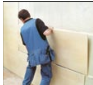
7 Fixing the next panel.
